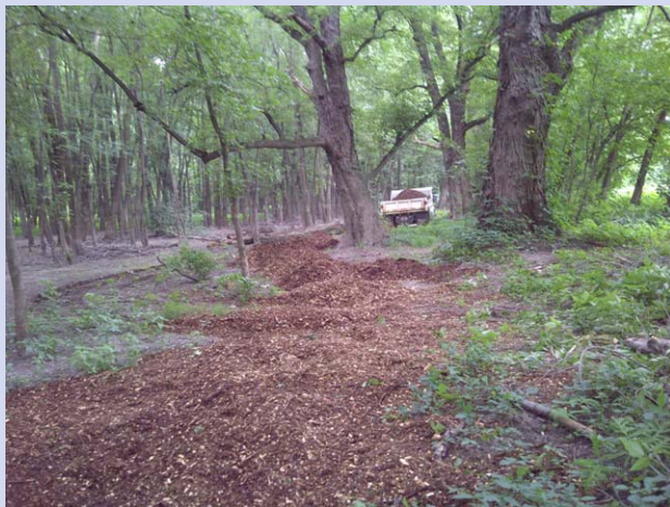
Community Court Community Service crews spreading wood chips on the new trail
