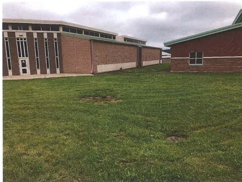
Photograph 4 – Building 4 (Left), Building 8 (Right)
